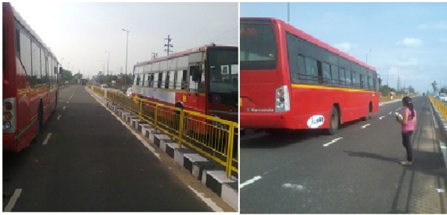
Fig. 6: Headway Survey is in Progress
